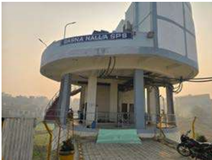
Picture 33 : Sewage Pumping Station over Basna Nala in Shantipuram, Phaphamau. Source: NIUA
