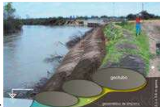
Geotubes for Embankment
