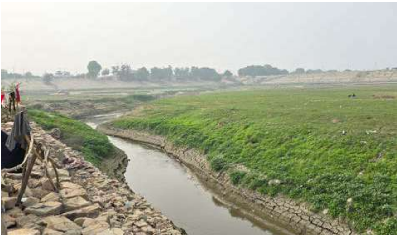
Picture 98: Drainage channel carrying treated wastewater from Salori STP to river Ganga, Source: NIUA
